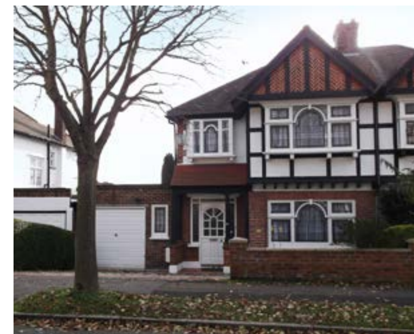
Figure 22: Decorative features at Sudbury Court
