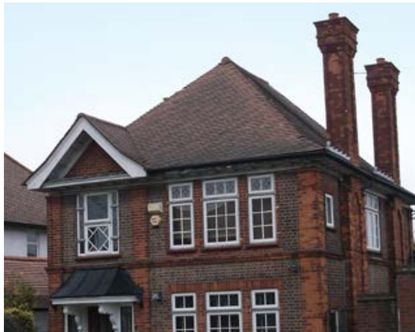
Figure 26: Decorative brick chimney at Sudbury Court
