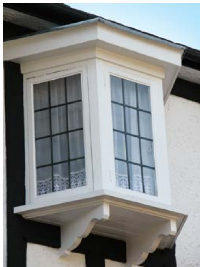
Figure 18: Window details at Sudbury Court
