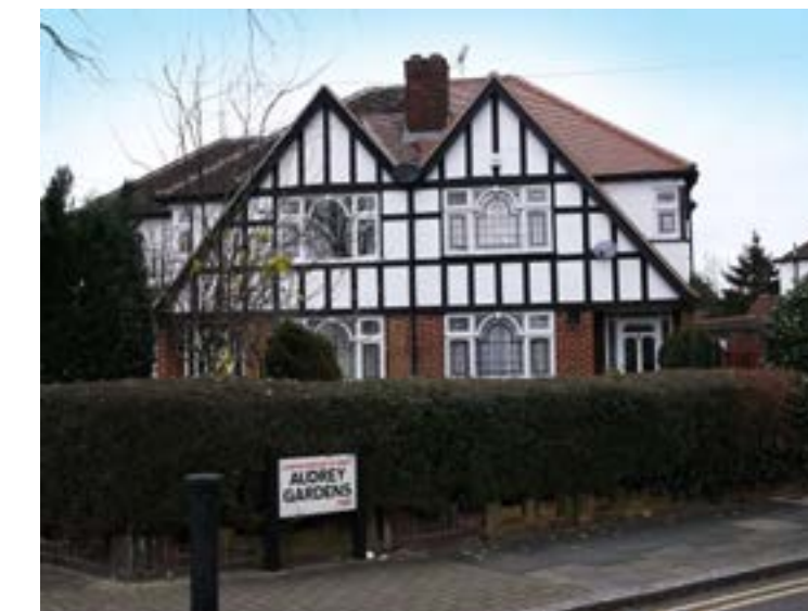
Figure 24: Half timbering at Sudbury Court
