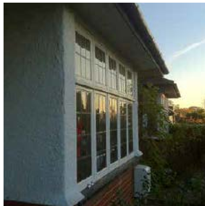
Figure 17: Window details at Sudbury Court
